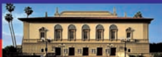
THE PASADENA CIVIC AUDITORIUM
